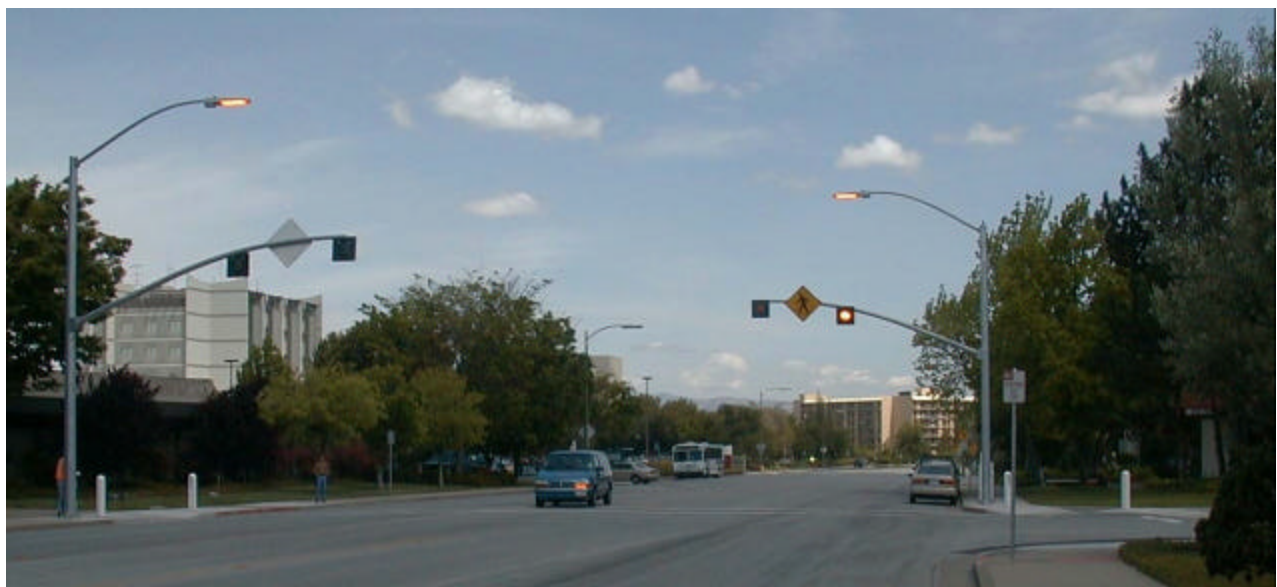
Figure 2: Samaritan Drive and Kinghurst Way standard overhead yellow flashing beacon
